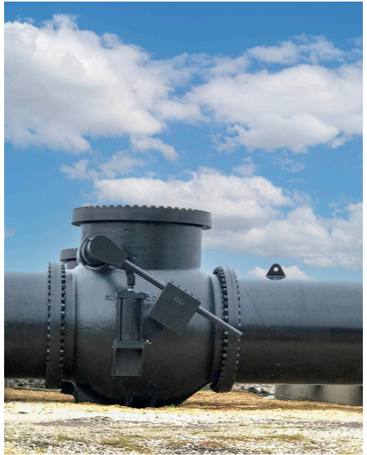
This 60" APCO Swing Check Valve is one of four that prevent the backflow of stormwater at the Louis Armstrong New Orleans Airport.
