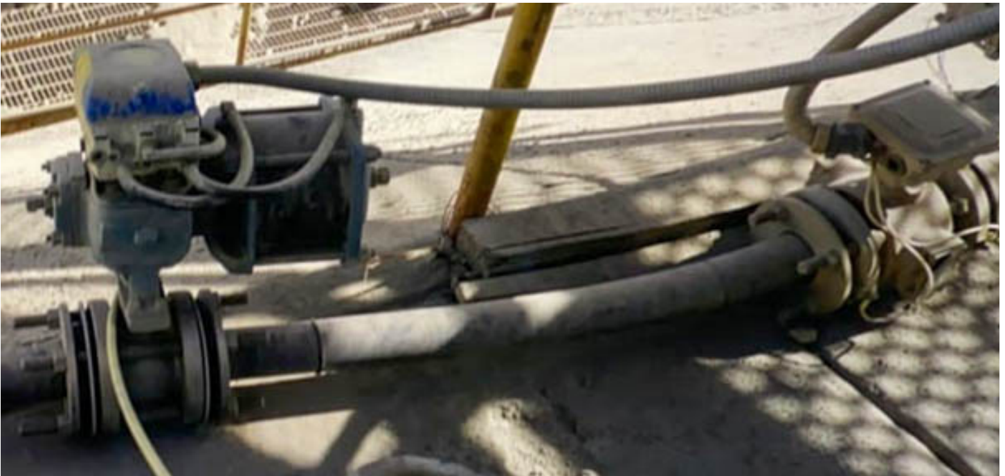
Raffinate Control - 2" RCV 317 stainless construction, full flow trim, PowerRac actuator, P201 positioner
