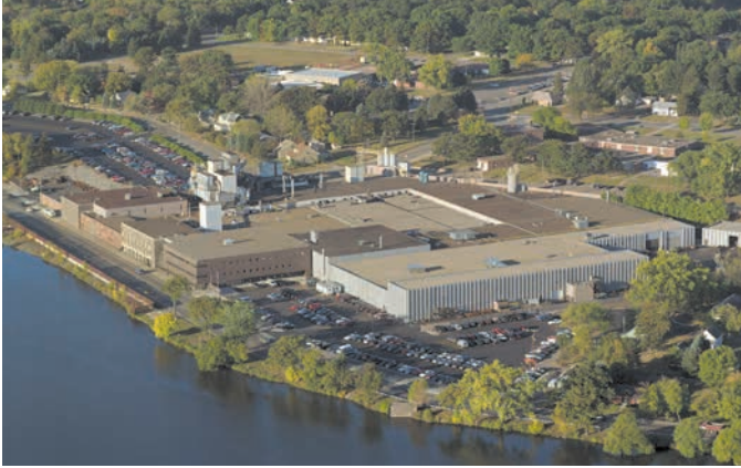
DeZURIK Corporate Headquarters and Manufacturing Facility, Sartell, MN, USA Established in 1928, 420,000 sq. ft.
